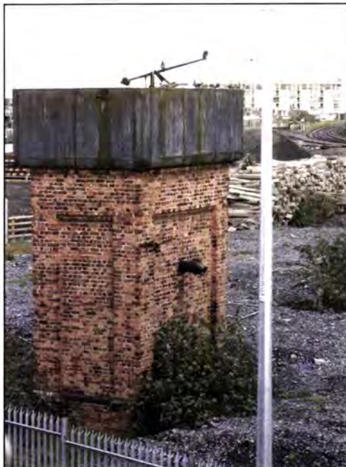
Plate 16: Water tower Sherriff Street Upper, Dublin
