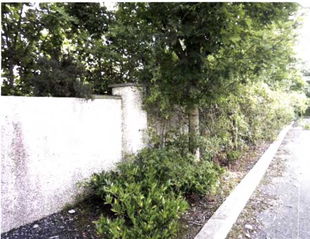
Photograph 4: Boundary wall separating Tesco car park to the west of the site
