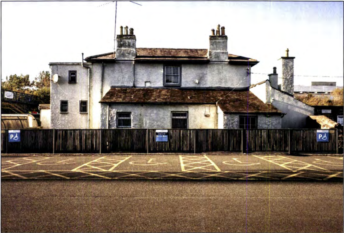
Plate 5: Arklow Station Rear Elevation, facing west.
