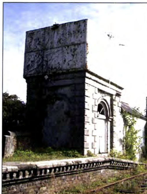
Plate 19: Rail water tower Moate Railway Station Co. Westmeath
