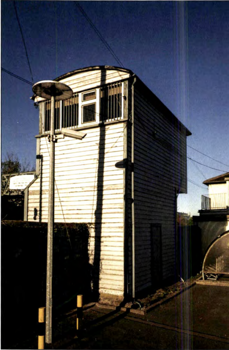
Plate 10: Signal box, facing northwest.
