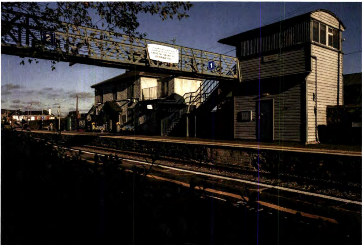
Plate 6: Footbridge and Signal Box, facing northeast.
