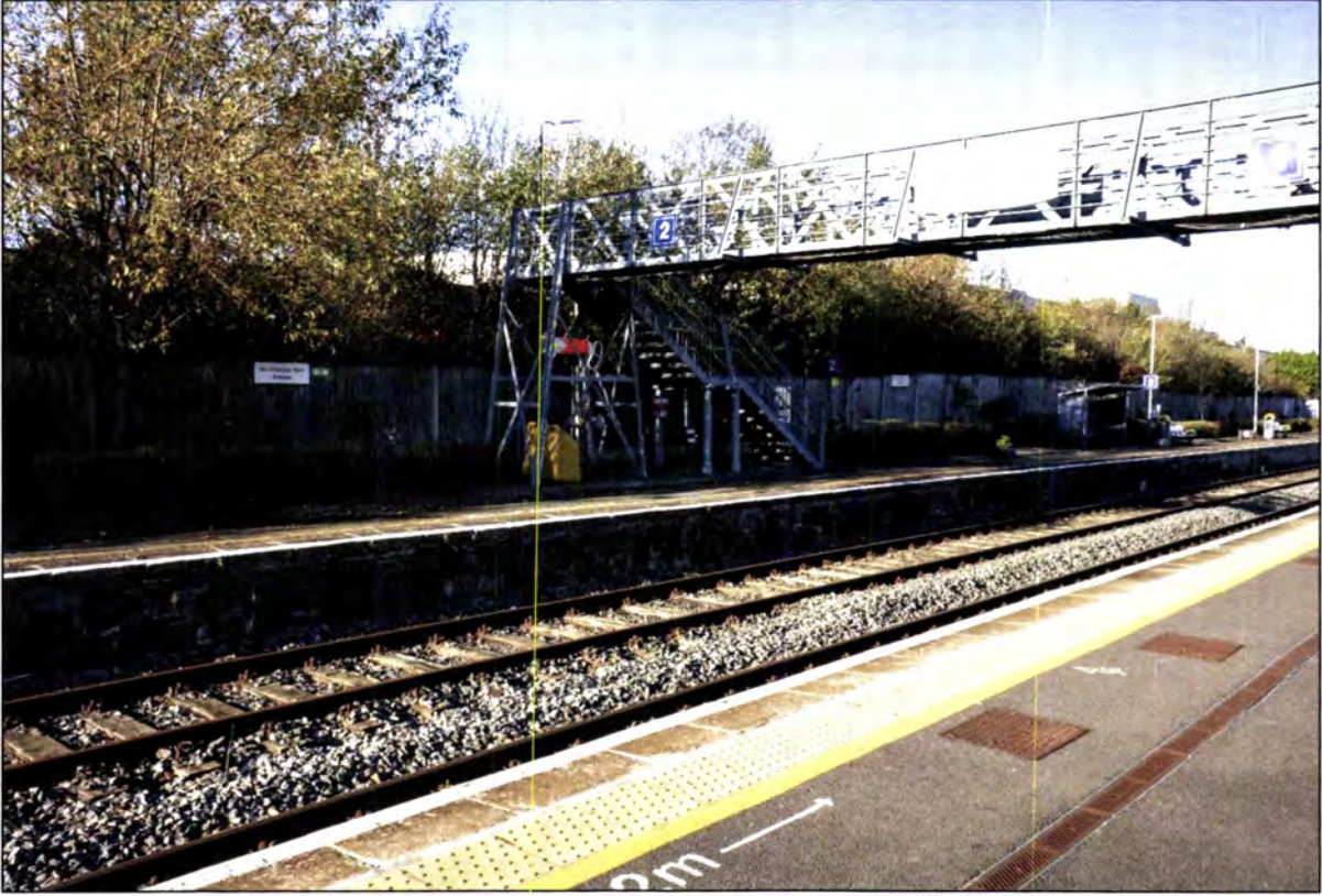
Plate 11: Footbridge looking northwest.
