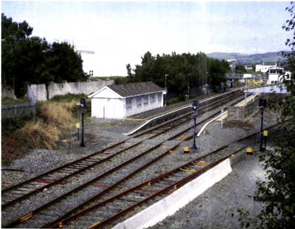
Photograph 1: Overview of station building
