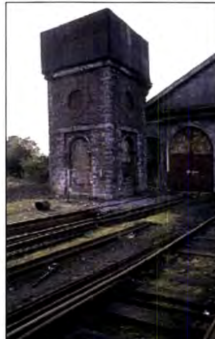
Plate 17: Water Tower, West Station Ranelagh, Dublin
