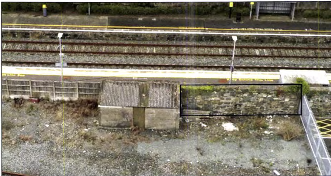
Figure 5 Section of masonry wall to be removed highlighted.
