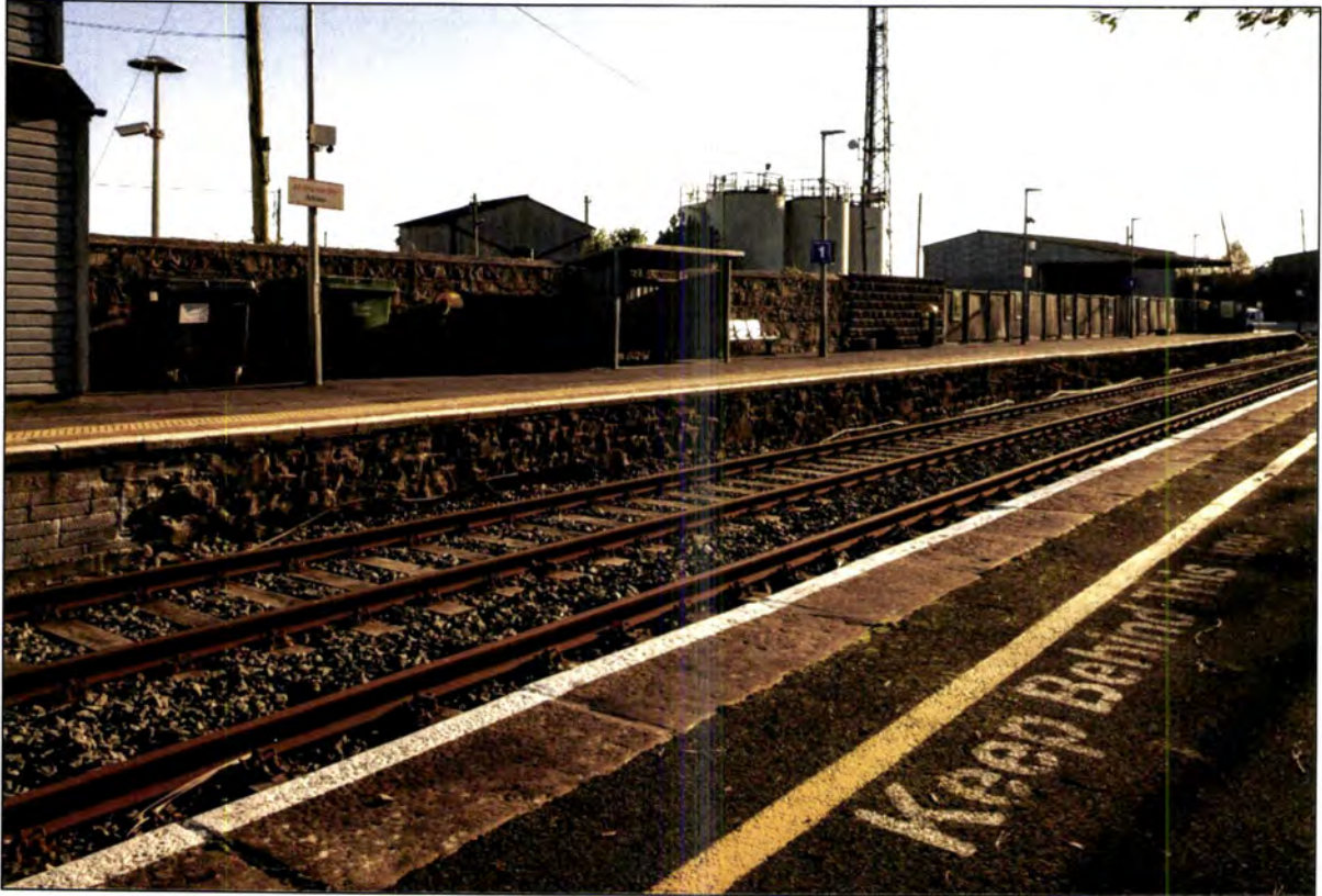
Plate 14: Looking southeast along east down platform, the southern bridge option would lie behind wall to right of shelter.
