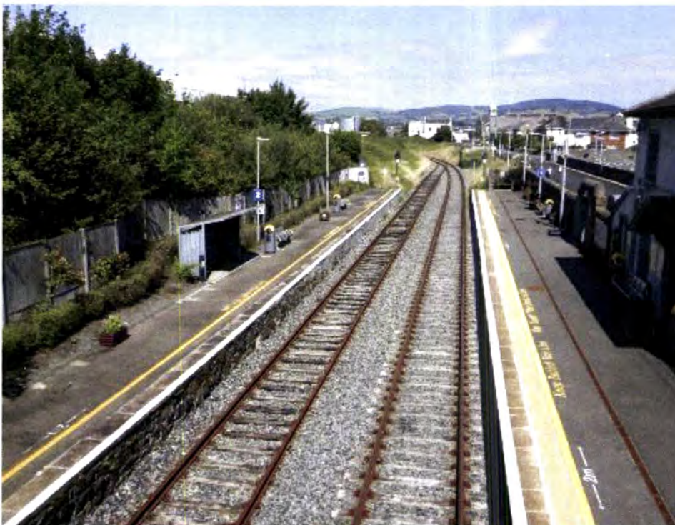
Photograph 2: Overview of platforms
